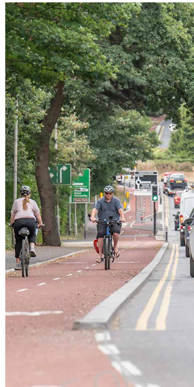
Delivering safer cycling facilities – segregated cycle lanes on Ringwood Road, Poole delivered through the Transforming Travel programme.
