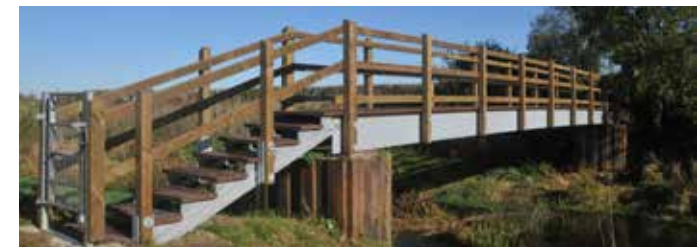
Refurbished footbridge in West Dorset improves pedestrian safety and supports active travel across rural infrastructure.
